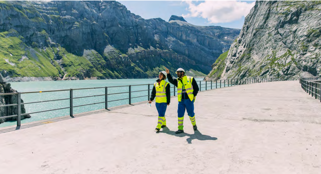
Hydro power stations, Linthal, Switzerland
