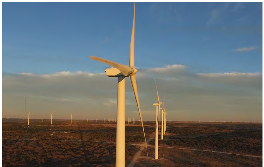
Wind farm in Texas, U.S.A.
